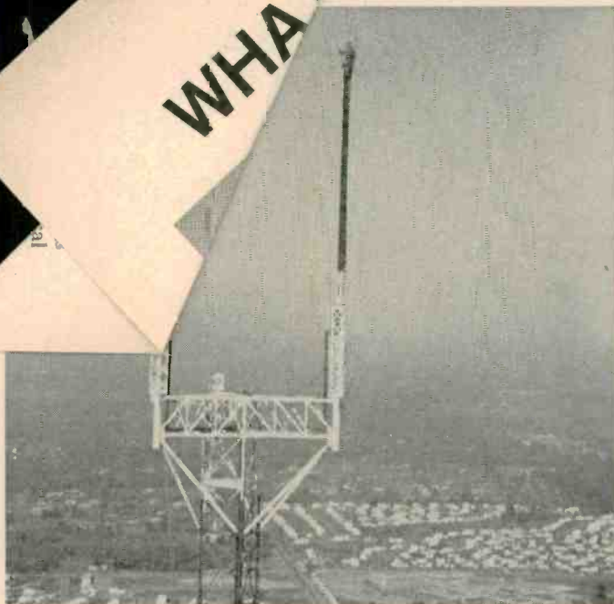
WORLD'S FIRST MULTIAN TENNA TOWER for uhf broadcasting stands 1,050 feet above Detroit area, where it's used by WKBD-TV and WTVS. WJMY-TV will add third antenna later.
